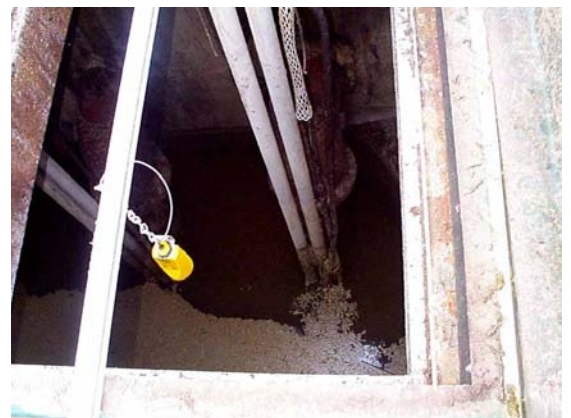
Mobrey DMSP900SH Ultrasonic Level Transmitter
